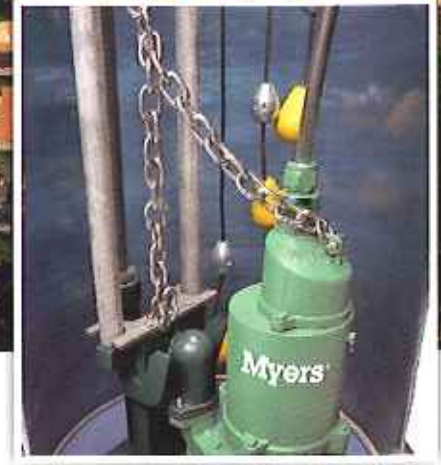
Lift-out rail system eliminates the need for personnel to enter the basin
